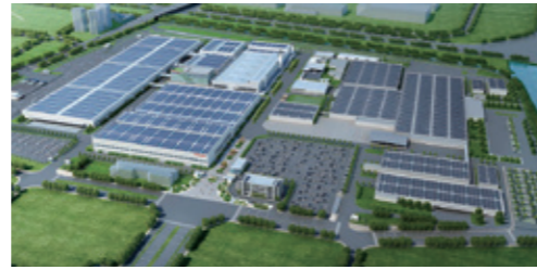
GAC Honda's new EV plant
