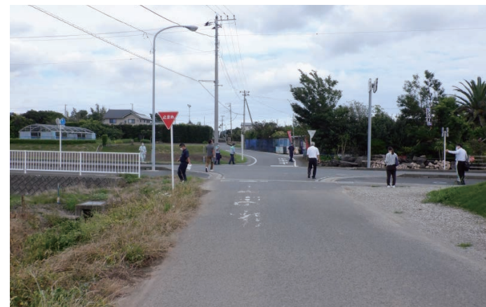
Before improvement: The "STOP" marking was fading.
