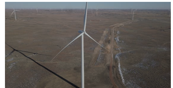
Boiling Springs Wind Farm (120 MW)
