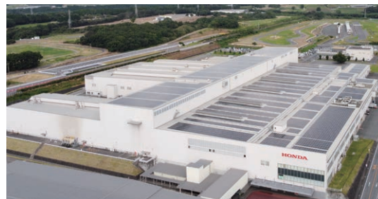
Kumamoto Factory (3.8 MW)
