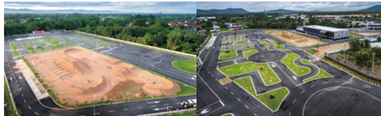
Traffic education facilities in Thailand (Chiang Mai (left) and Phuket (right))
