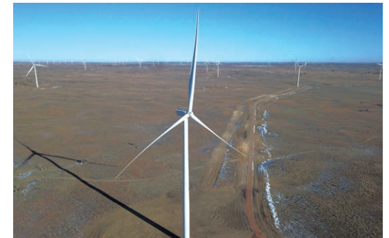
Boiling Springs Wind Farm (120 MW)
